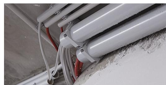
Thanks to the functional clip system, several EC Euro clips can be clipped together in various sizes.
